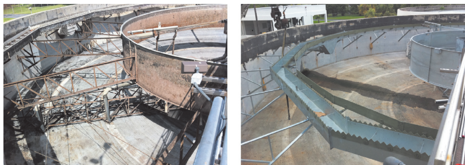
Figure 7. Original (left) and Retrofitted (right) Influent Center Well
