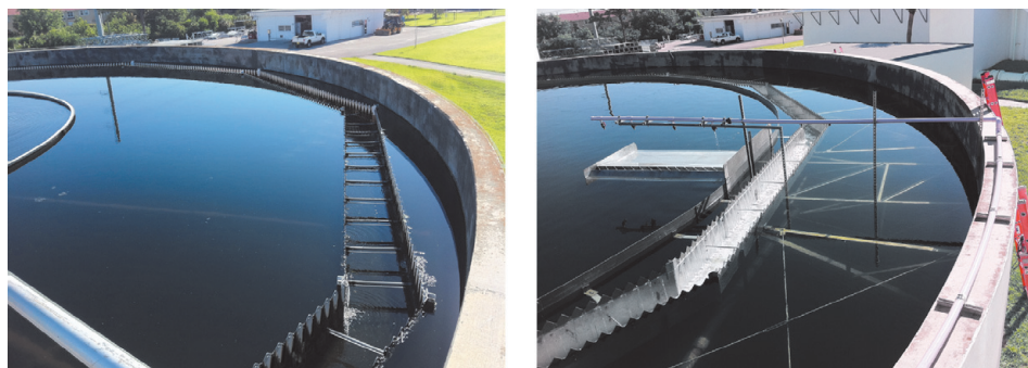
Figure 6. Original (left) and Retrofitted (right) Effluent Launder
